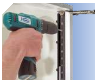
Drilling for placing shelves.
