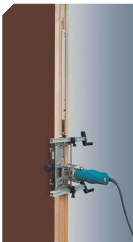
Making the second recess on the frame.
